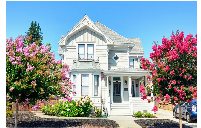
View of an historic single family house in the Fuller Park neighborhood.
