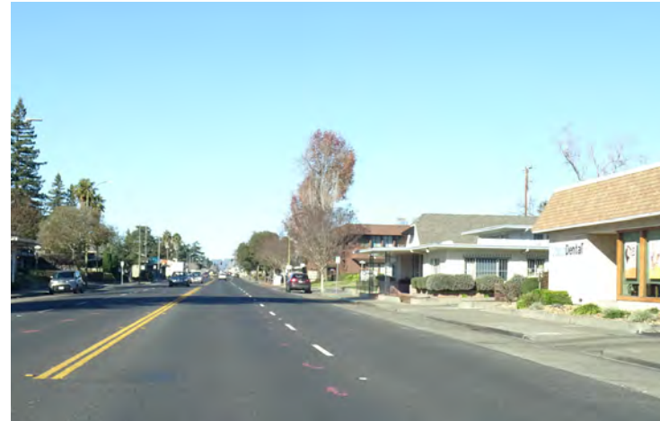
View of the existing streetscape along Jefferson Street near F Street
